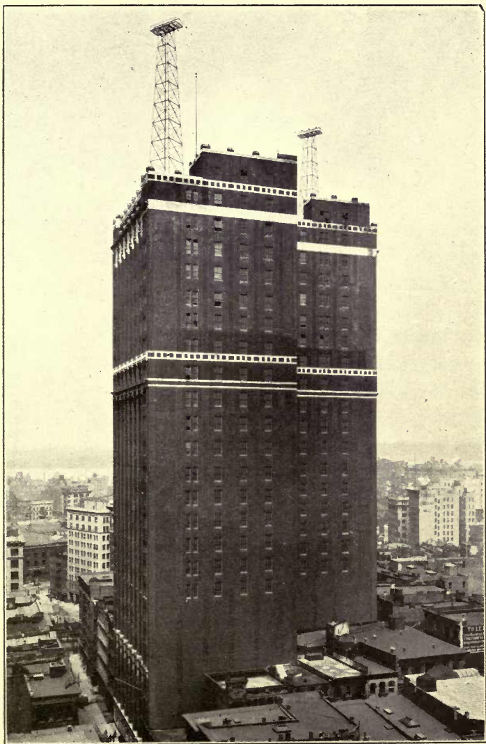
PL. XII.—BROADCASTING STATION OF THE AMERICAN TELEPHONE AND TELEGRAPH COMPANY ON THE ROOF OF THE WALKER-LISPENARD BLDG. IN NEW YORK CITY WHERE THE LONG-DISTANCE TELEPHONE LINES TERMINATE.
